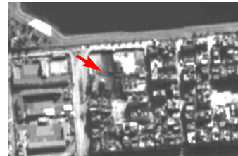
2. Buildings: Severely Damaged
